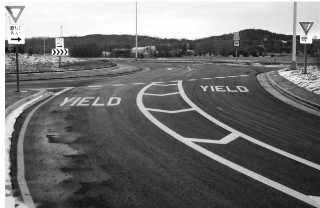
Figure 2-16b: Occasional entry with double white lines separating entry lanes. STH 35 and Hanley Road near Hudson.
